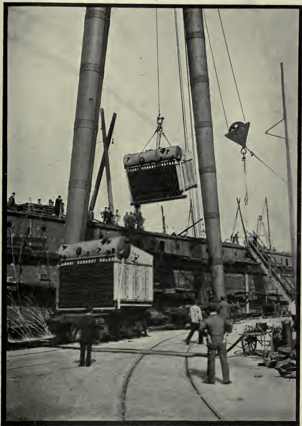
HOISTING WATER-TUBE BOILERS ON BOARD.
