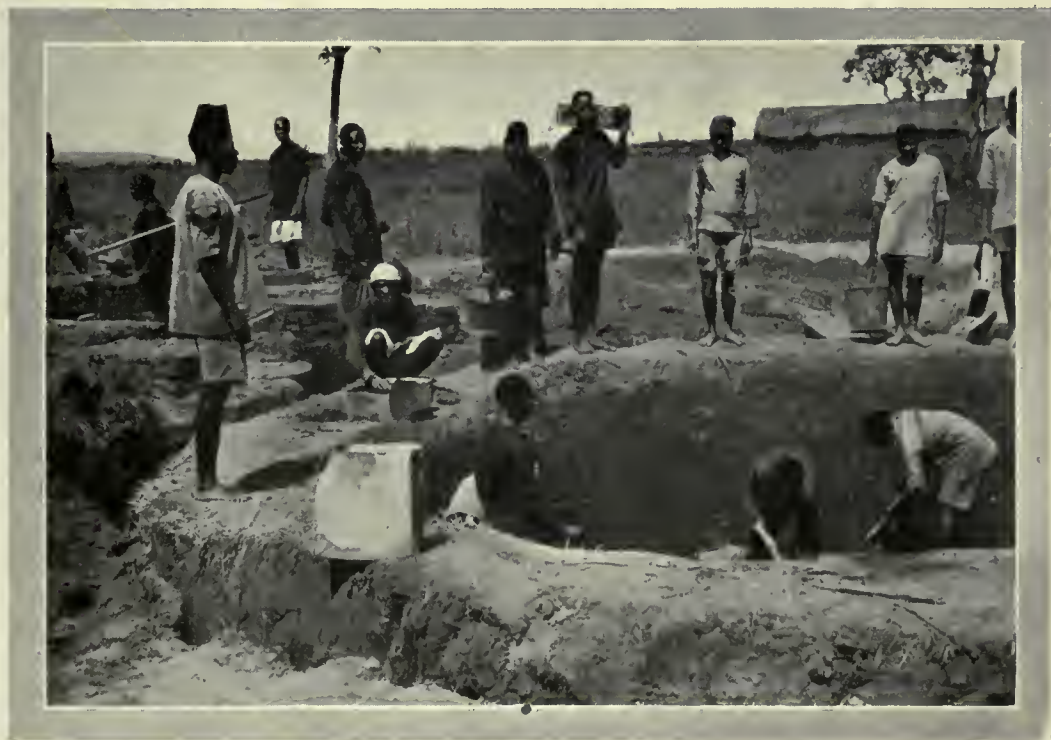
BUILDING A BLOCKHOUSE.
