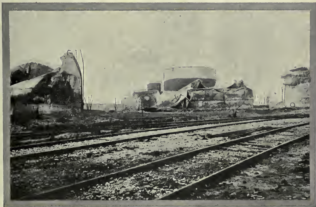
REMAINS OF OIL TANKS AT FLOESHTI DESTROYED BY THE BRITISH.
