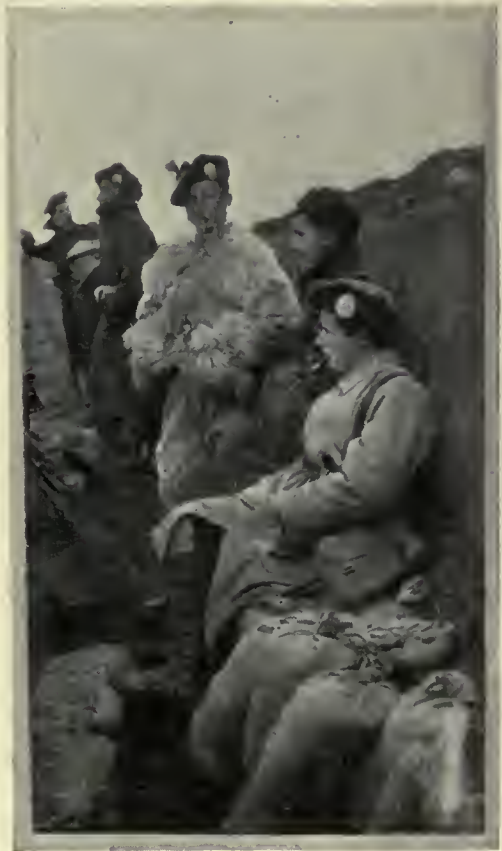
WINTER IN THE TRENCHES.
