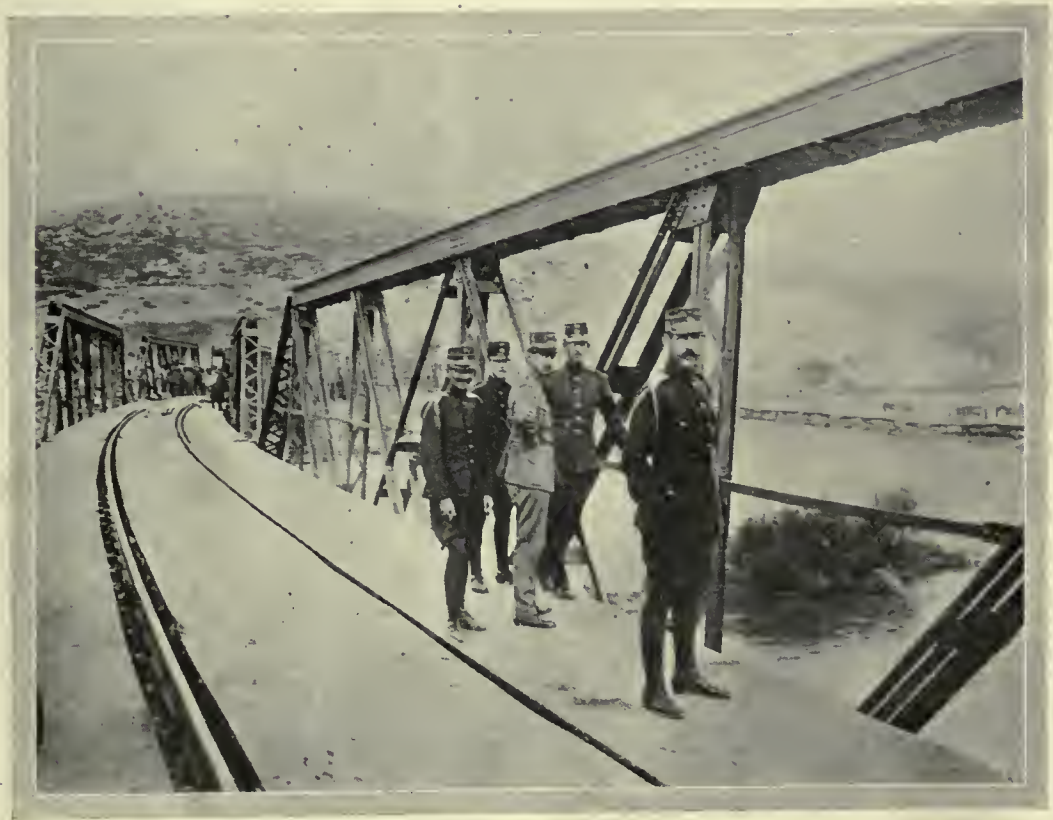
THE RAILWAY VIADUCT OVER THE STRUMA AT DEMIRHISSAR, Destroyed by the Allies in order to interrupt the communications between Bulgarian and Turkish forces.
