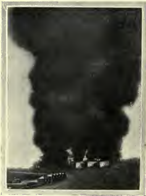
AN OIL-WELL IN RUMANIA, SET ABLAZE BY THE BRITISH.
