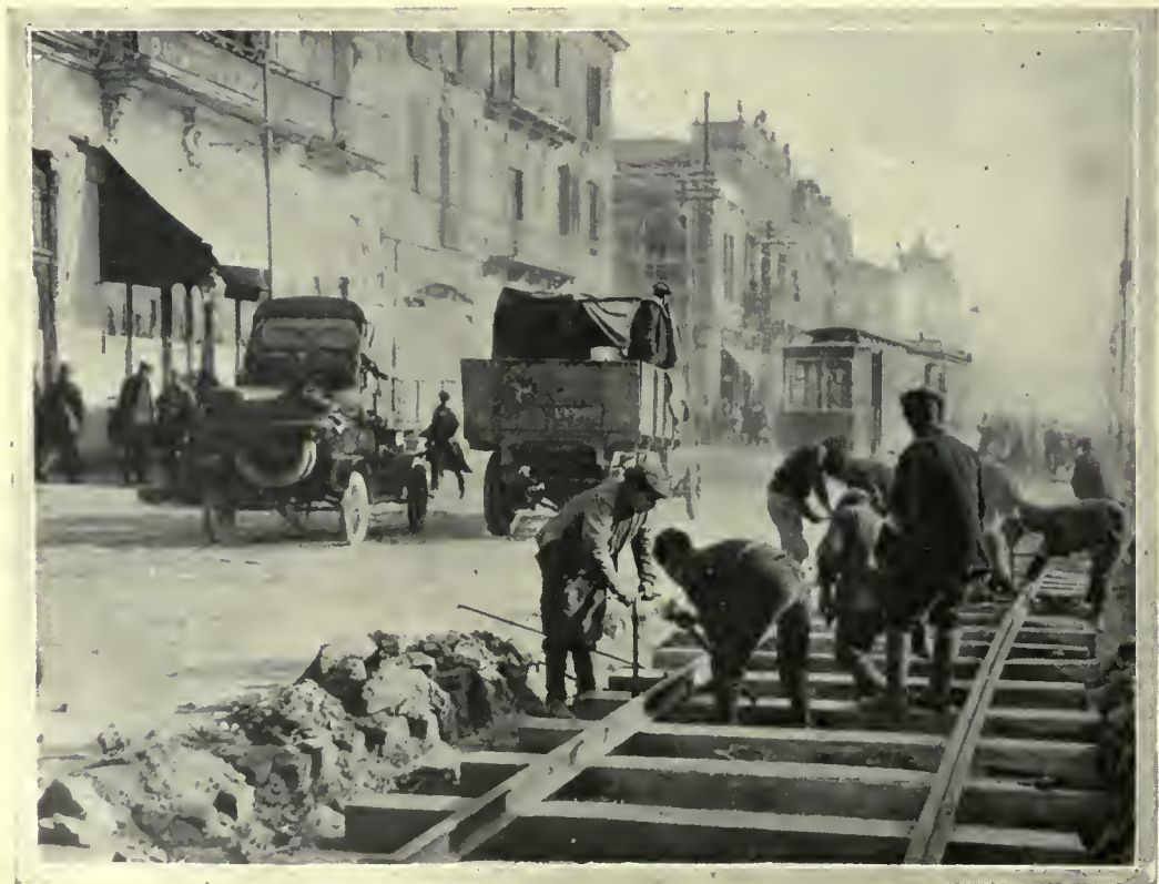
LAYING A RAILWAY THROUGH SALONIKA.
