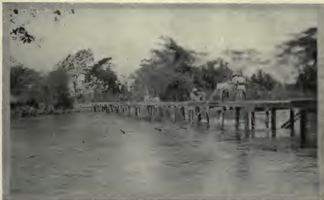
BRIDGE OVER THE PANGANI AT MIKOTSHENI.
