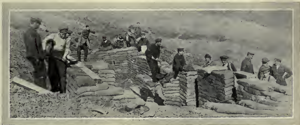
BUILDING A SANDBAG VILLA ON THE HILLS.
