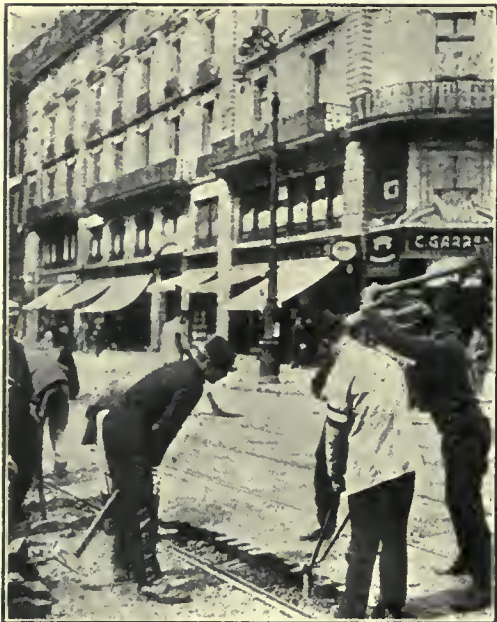
FRENCH PRISONERS REPAIRING THE TRAM LINE IN FRANKFORT.
